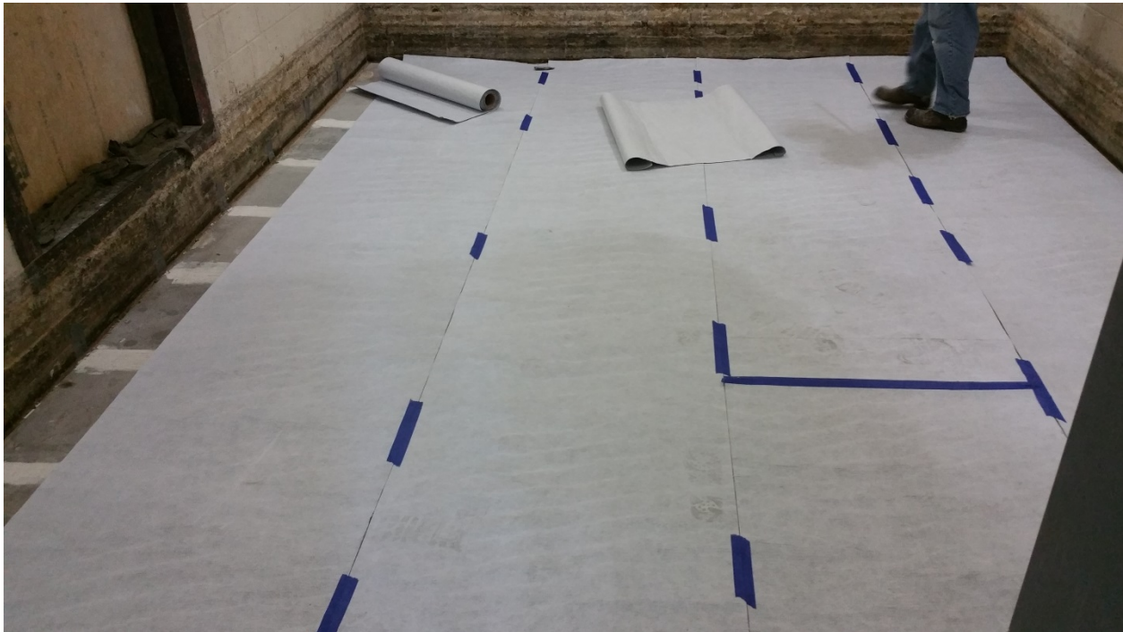
Figure 2 – Fracture Ban™ 90 membrane placed over concrete slabs.
